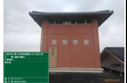
避雷針施工前
